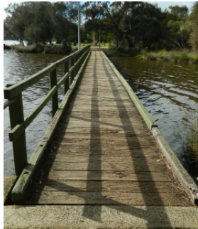
bridge over Collie River to Watson Acceptance Carol Armstrong
